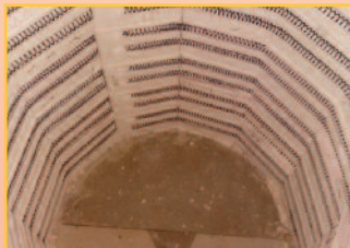
Before & After replacement of a top loading kiln element set: Note the essential repair of the burnt out hot spot!
